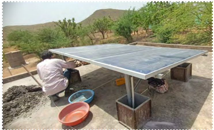
Solar Panel installation
